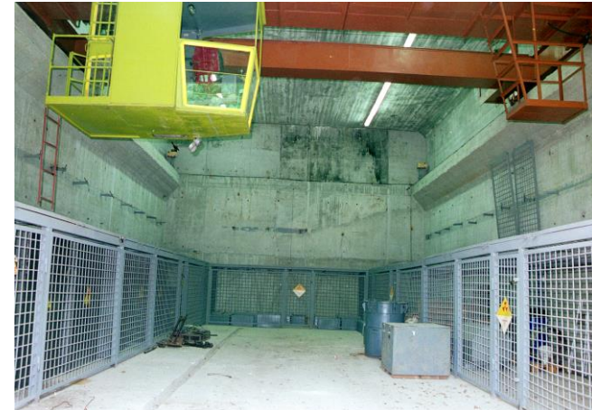
Picture 4. Inside of Surface storage from armed concrete
