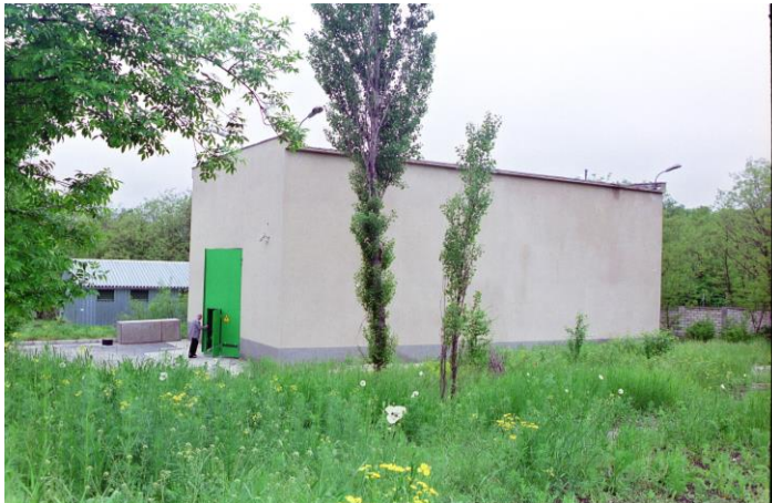
Picture 3. Surface storage from armed concrete
